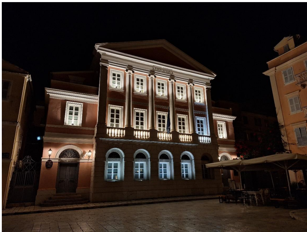
Building of the Banknote Museum of the Ionian Bank – Alpha Bank ©Annika Heinze, State Agency for Civic Education Rhineland-Palatinate
